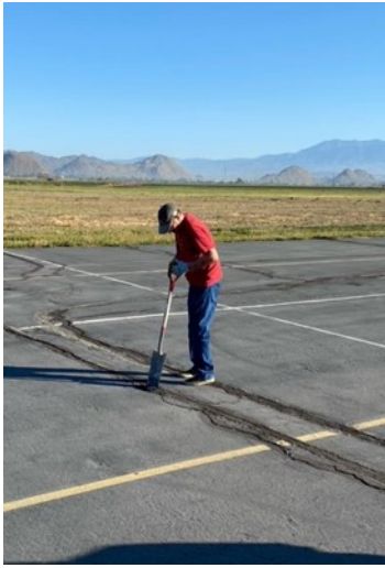
Dave Kennedy filling cracks.
