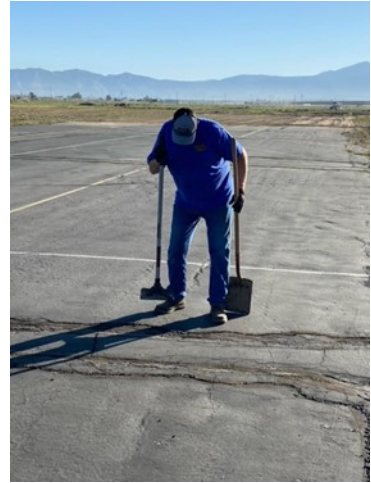
Jim Layes filling cracks.
